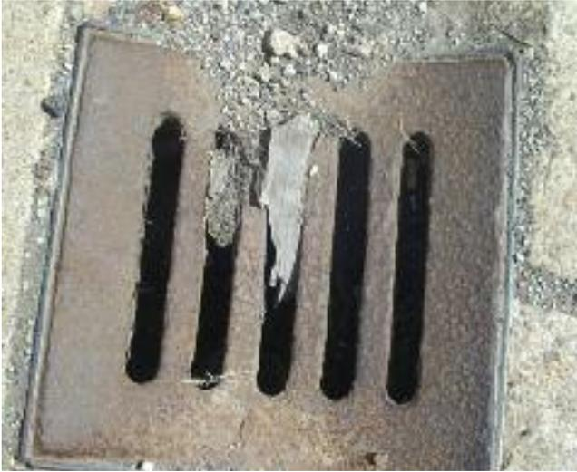
**Cleaning and maintenance:** Drainage systems need regular maintenance to make sure that they work properly. Clean gullies regularly to remove the debris that collects in them. Cracked and broken pipes should be repaired and roots removed. You could use specialist drainage contractors to do this, or your local council may provide this service.
